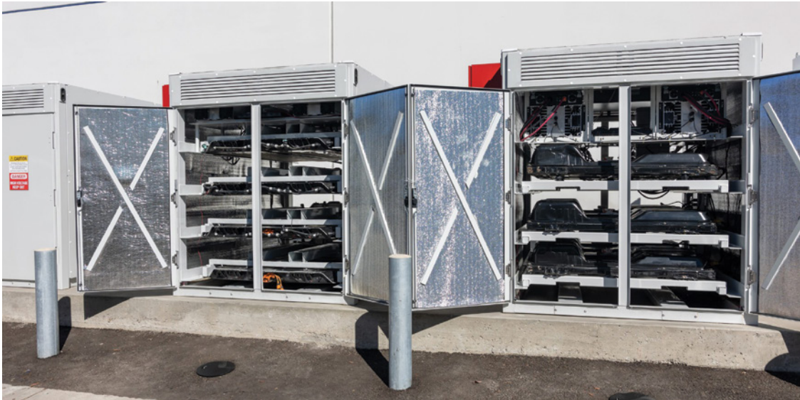
FIGURE 11.2 Advanced battery-management systems being used as stationary storage capacity
