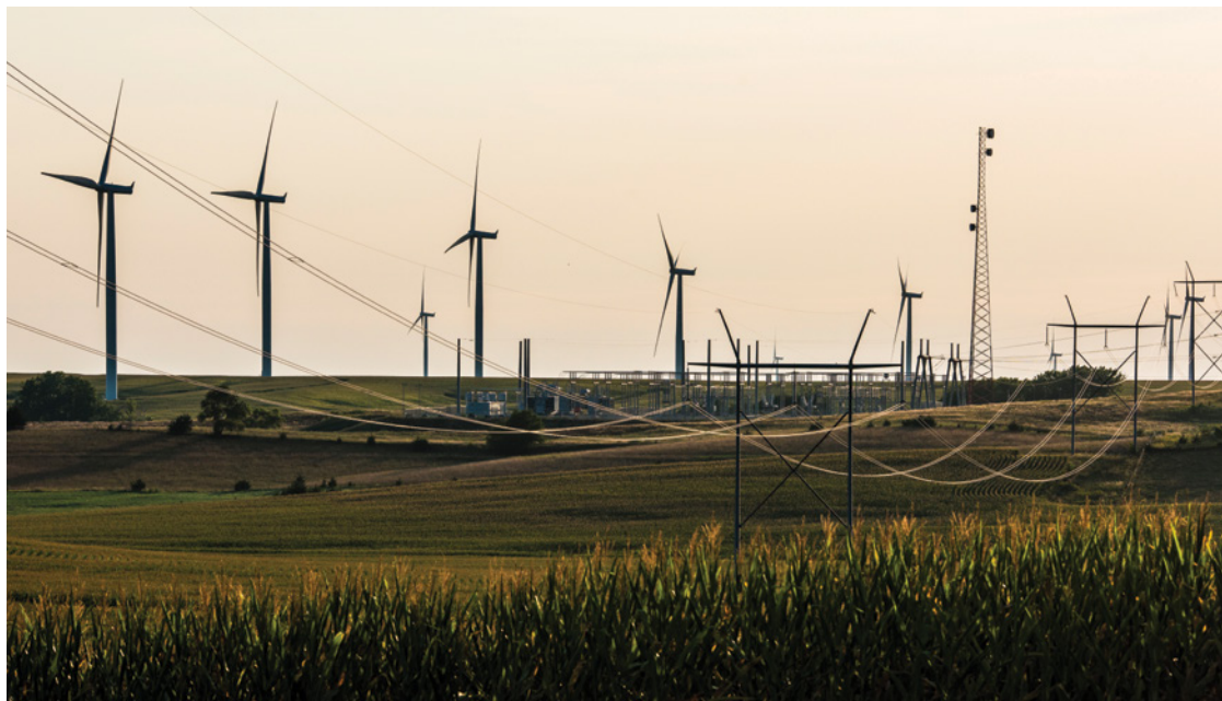
FIGURE 10.5 A cluster of wind turbines
